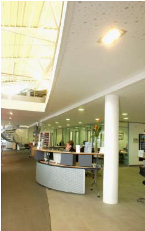
One of the Four Interact Fire Solutions Fire Protected Columns
